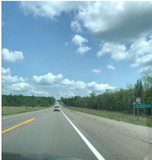
US-2 (Iron County): 8-foot paved shoulders with rumble strips reducing rideable width (image courtesy of WUPPDR)
