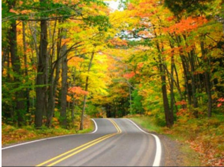
US-41 (Keweenaw County) north of Delaware (Bete Gris Road) has no paved shoulders
