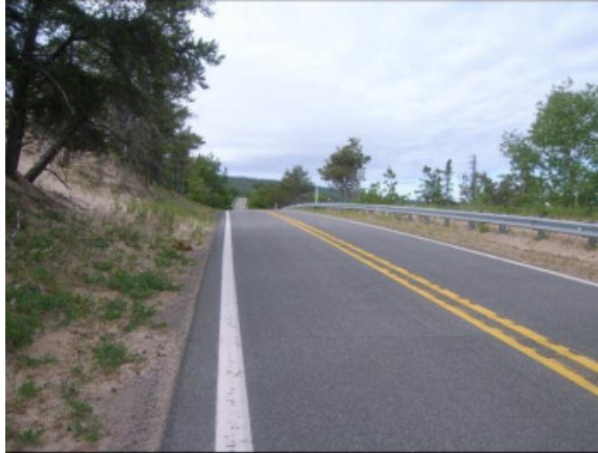
M-26 near Great Sand Bay between Eagle River & Copper Harbor has no paved shoulders (photo courtesy of WUPPDR)
